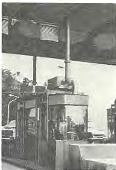
図 10. 空調機とダクトの設置状況 Duct and the air conditioner set up.
