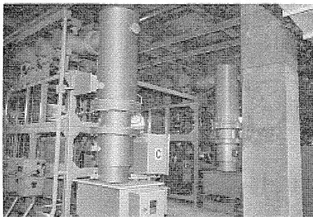
図 3.1 関西電力(株)新曽根崎変電所納め 154 kV ガス絶縁開閉装置 154 kV gas insulated switchgear installed at Shinsonnezaki substation of Kansai Electric Power Co.
