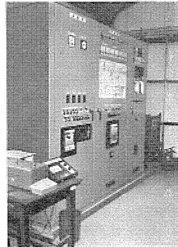
図 2.12 制御盤 (左の2盤, 右端は受電盤) Control boards (two boards on the left one board on the right is incoming board).
