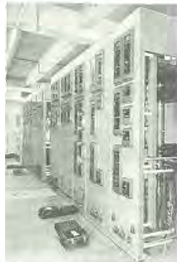
図 2.2 新六甲変電所配電盤 (保護継電盤) Switchboard of substation (protection relay panel)
