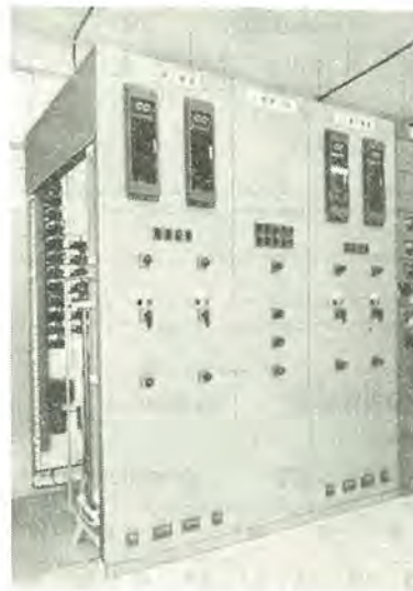
図 2. 6 補助き電区分所配電盤前面 Switchboard of sub-sectioning post (front view).
