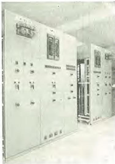
図 2. 5 き電区分所用配電盤 Switchboard of sectioning post.
