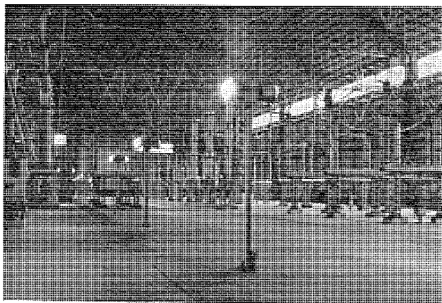
図6.1 275 kV 特高開閉所の照明 Illumination of 275 kV extra high tension switching station.
