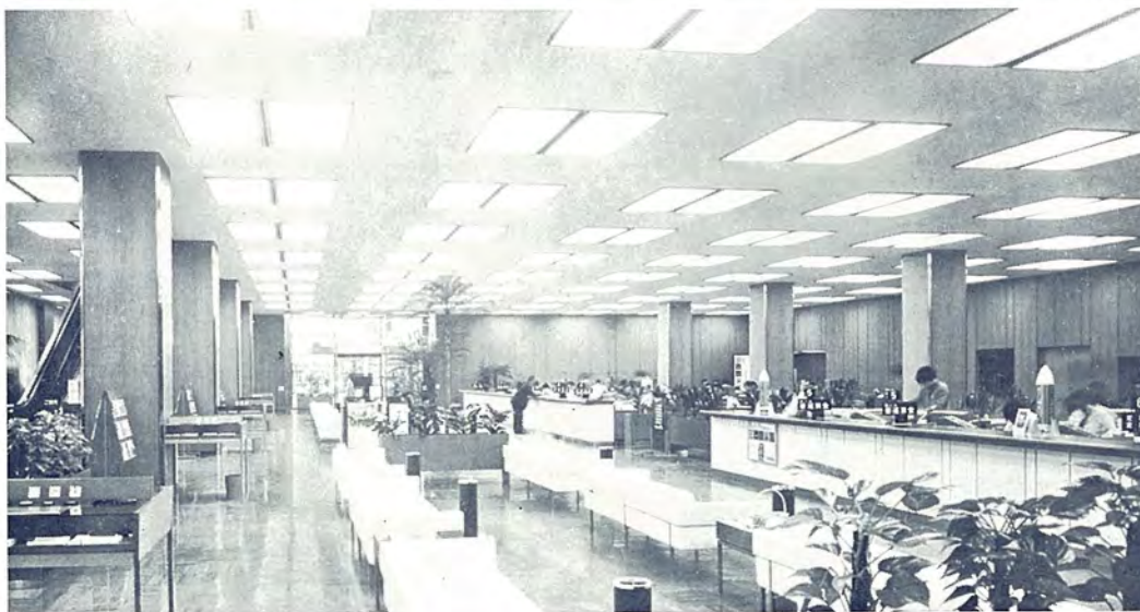
八十二銀行本店営業室 (長野) 空調形けい光灯40W×8灯 ×2台×99台 初期照度 2,000 lx Business room of Hachijuni Bank Head Office Nagano Prefecture Airconditioned type fluores- cent light 2×8×40W lamps total 99 sets
