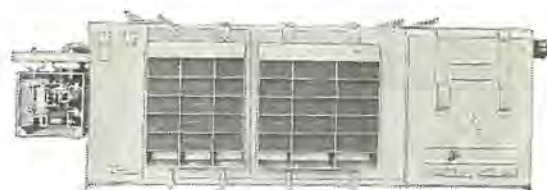
図 7. 1 HB-8 R-643 形断流器箱外観 Type HB-8 R-643 line breaker box.
