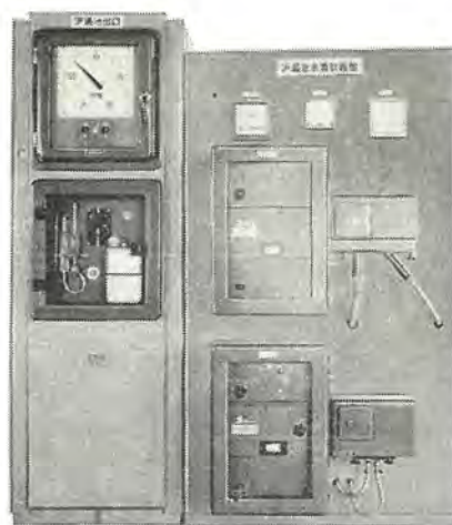
図 4.8 ろ過池水質計器盤 Instrument panel for quality of water sampled from filter bed.
