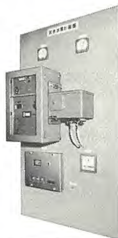
図 4.9 送水水質計器盤 Instrument panel for quality of clean water.
