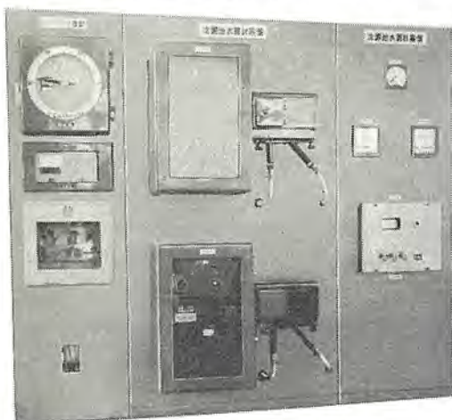
図 4.7 沈殿池水質計器盤 Instrument panel for quality of water sampled from sedimentation tank.
