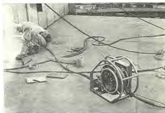
図 5.7 造船現場での溶接 (その 1) Welding for fabricating work in the ship-building yard.
