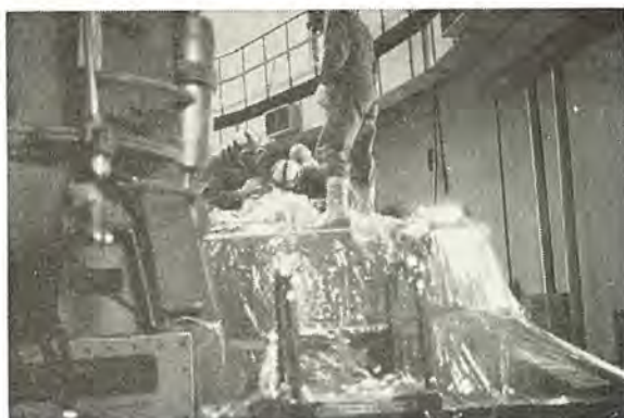
図 2.3 溶接状況 Fig. 2.3 Welding operation.
