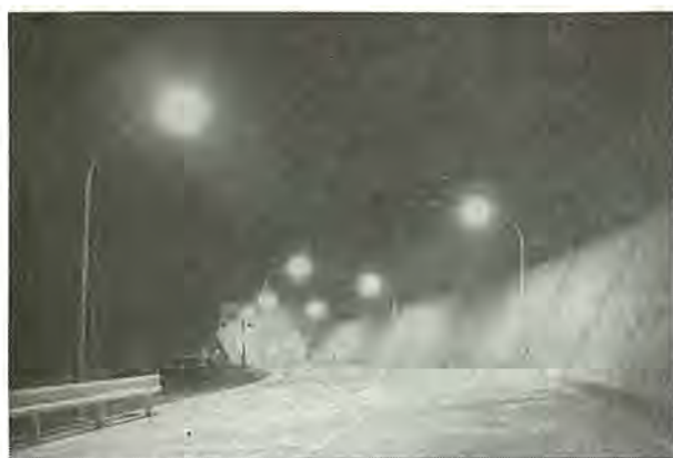
図 3.6 入口部の夜間緩和照明の状況 Fig. 3.6 Lighting at night at the entrance of tunnel with consideration of relieving sudden change of brightness.
