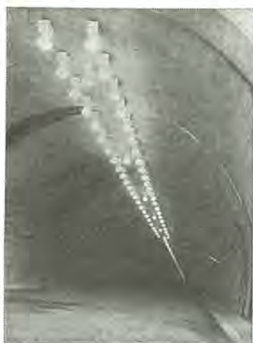
図 3.5 増灯緩和照明器具の配置状況 Fig. 3.5 Arrangement of increased luminaires for relieving sudden change of brightness in the tunnel.
