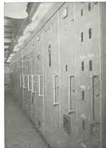
図3.2 (b) VA-C形船用配電盤外観 Fig. 3.2 (b) Exterior view of switchboard for marine use.
