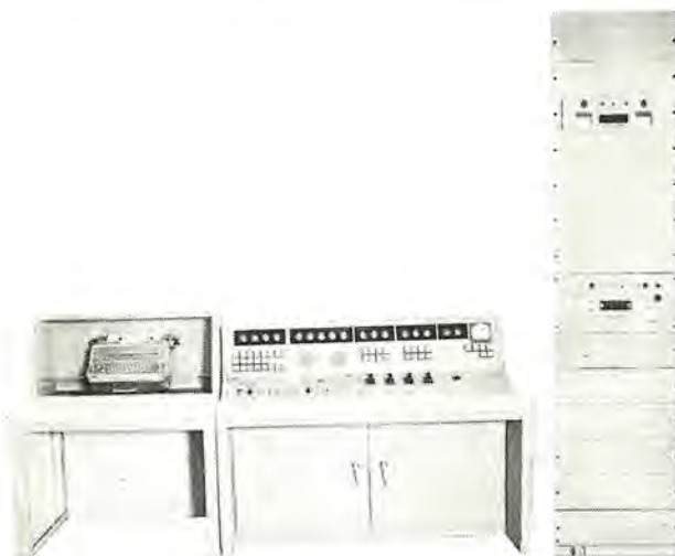
図 11-27 テレメータ放流警報監視制御装置 Supervisory and control equipment of telemetering and flow alarming system.
