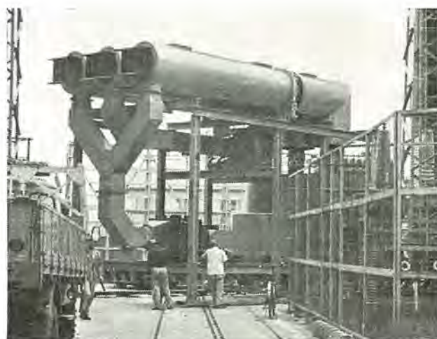
図 2-59 17,000A 強制空冷式 離相母線 17,000A forced air cooling isolated phase busduct.
