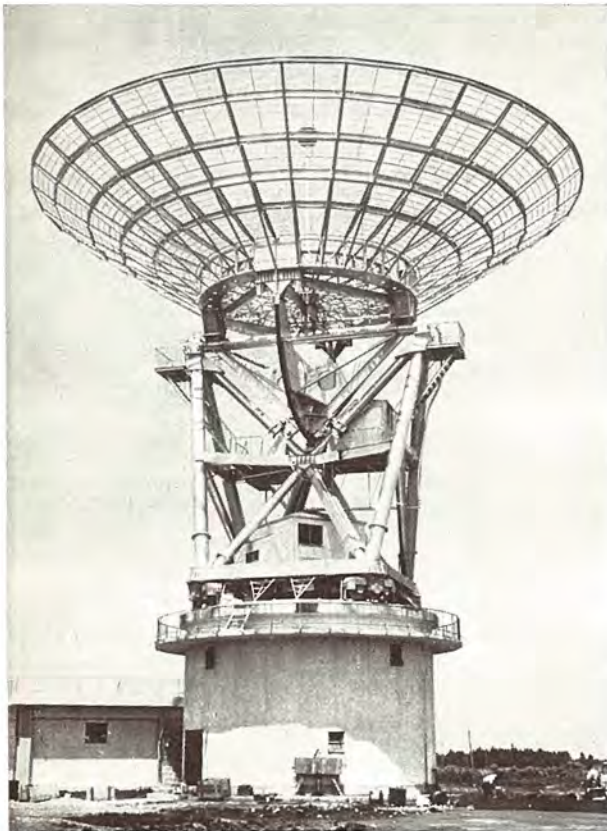
VHF 遠距離レーダ用空中線装置 25 meter experimental antenna for long range radar and radio physics research.
