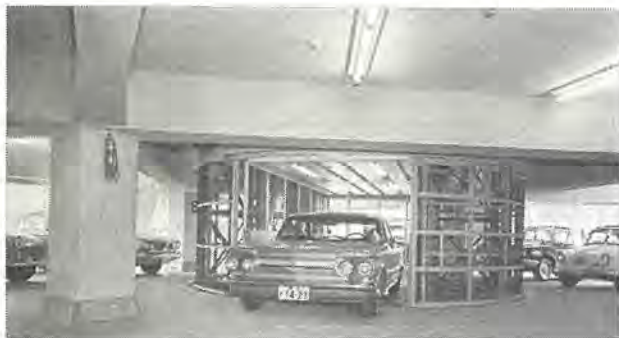
図 4.7 中川ビル駐車場一般階全景 Fig. 4.7 Full view of 1st floor parking place, Nakagawa Bldg.
