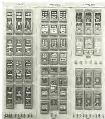
図 1.1 PC-337 形搬送保護継電装置 Fig. 1.1 Front view of carrier protective relay panel.
