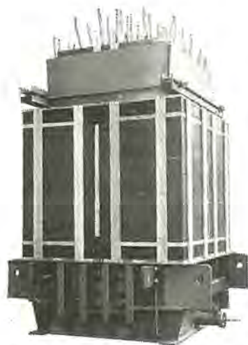
図 3.12 高圧短絡変圧器中身 Fig. 3.12 Core and coil assembly.
