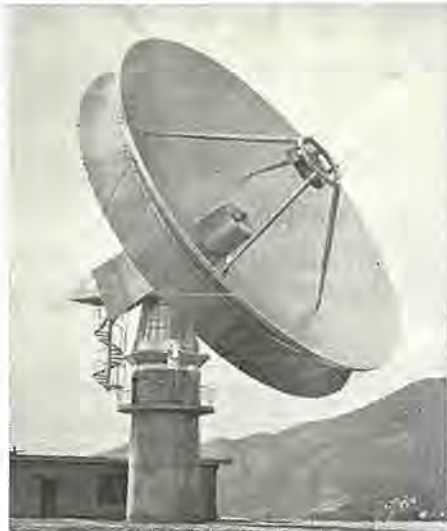
図 2.1 空中線装置および油圧室 Fig. 2.1 Close-up view of 18mφ tracking telemeter antenna and hydraulic power room.
