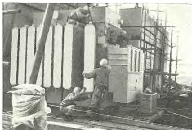
図 4.9 変圧器の組立作業中 Fig. 4.9 Main transformer in assembling.
