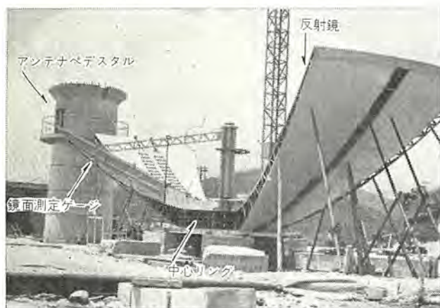
図4.2 反射鏡組立 Fig. 4.2 Construction work of 18m \phi antenna.
