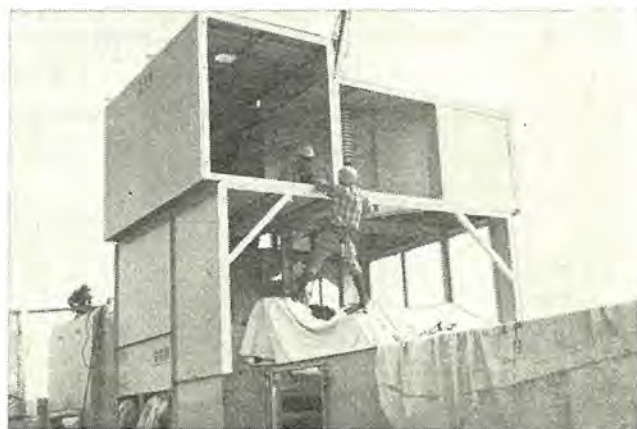
図4.4 ワッ組立作業中 Fig. 4.4 Cubicle frames in assembling.
