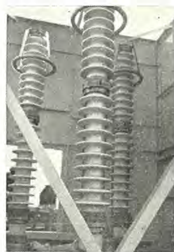
図 4.10 避雷器組込状態 Fig. 4.10 Setup of lightning arresters.
