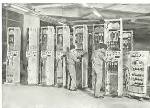
図 11-14 基地局受信架の試験 Inspection of receiver bay of repeater station.
