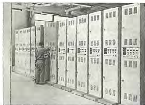
図 11-13 基地局送信架の試験 Inspection of transmitter bay of repeater station.
