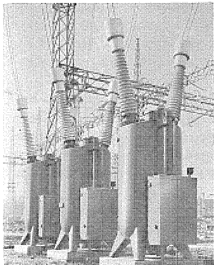
図 2.2 300 kV 15,000 MVA 2,000 A 油シヤ断器 (250-GW-1,500) Fig. 2.2 300 kV 15,000 MVA 2,000 A oil circuit breaker.
