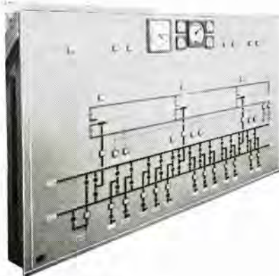
図 2-42 新しい照光盤 Appearance of new illuminative mimic bus.
