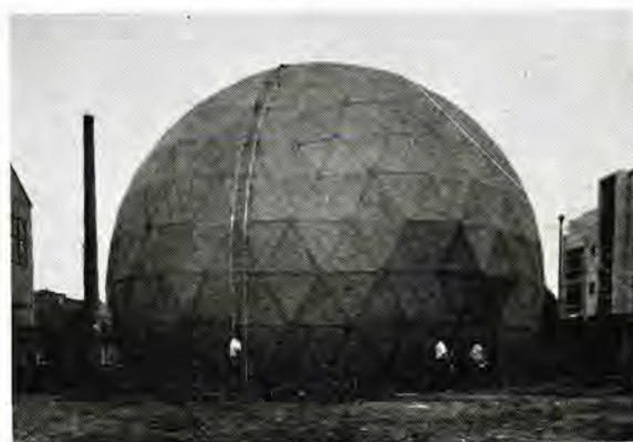
図 11-47 硬質ラドーム NCW-6/GPS Rigid reinforced plastics radome NCW-6/GPS.
