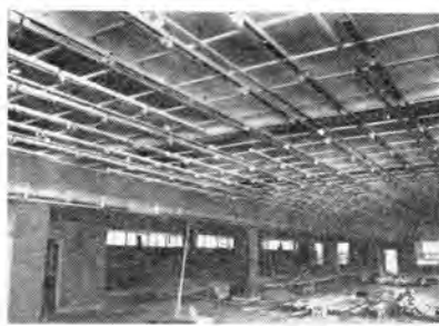
図 7.4 ケイ光灯器具を連続に取付ける Fig. 7.4 Fluorescent lamp of continuous mounting.
