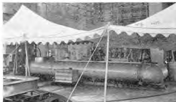
図 3.1 強制冷却の実験用母線設備 Fig. 3.1 Forced air cooled bus for testing.
