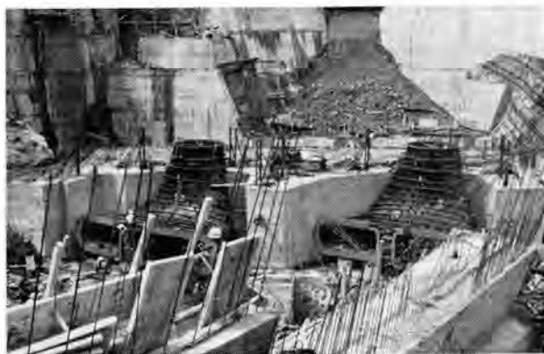
図 3.11 現地すえ付中の吸出管 Fig. 3.11 Draft tube under assembling at the site.
