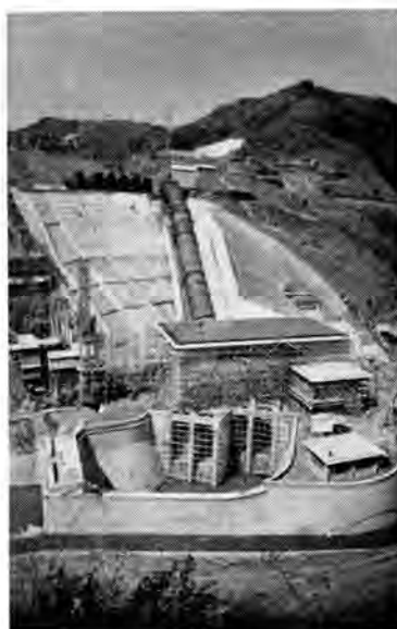
図 3.12 建設中の発電所全景 Fig. 3.12 Panoramic view of the power station under construction.
