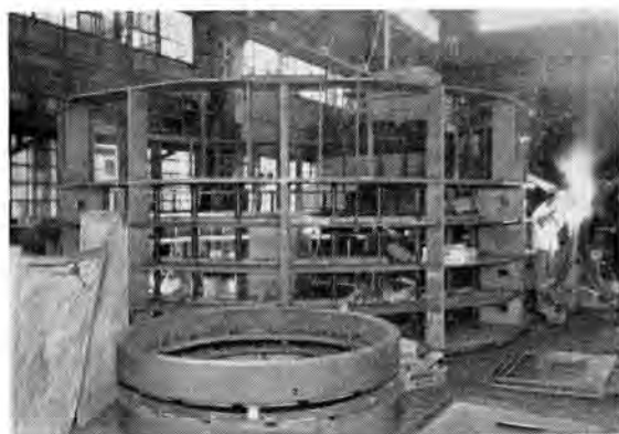
図 3.4 溶接中の固定子ワ Fig. 3.4 Stator frame under welding.
