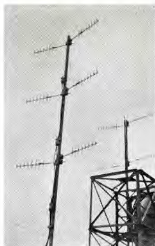
図 3.12 米原基地局送受信空中線 Fig. 3.12 Transmitting and receiving antennas of Maibara base station.
