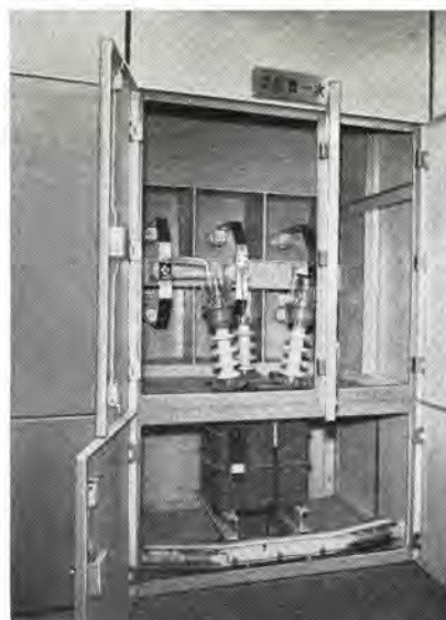
図 3.7 計器用変圧変流器のキュービクル状態 Fig. 3.7 Set-up of cubicle for potential and current transformers.
