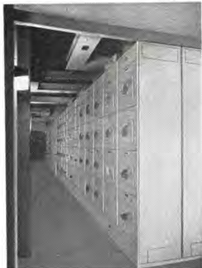
Fig. 3.2 Type NC-2300 B control centers on the second floor of the underground substation. (rear side)
