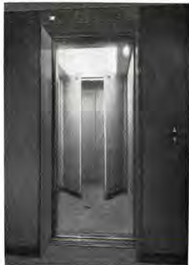
図 3.1 東2号機のカゴ室奥の間仕切を開いたところ Fig. 3.1 Car of East No. 2 with the partition at its further end left open.
