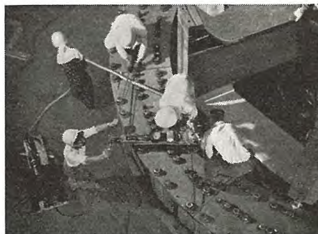
図 III. 3.2 回転子リム積 (ギヤドレンチによる締付) Fig. III. 3.2 Building the spider rim (tightening reamer bolts with geared torque indicating wrench).
