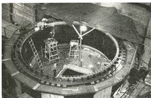
図 III, 2.1 固定子巻線 (コイル入れ作業) Fig. III. 2.1 Stator winding (Inserting stator coils into slots).
