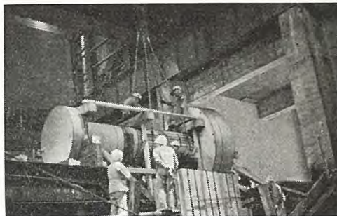
図 III. 1.3 発電機軸の荷おろし Fig. III. 1.3 Transportation of generator shaft.
