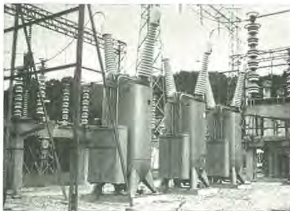
250-GW-500T 形油シャ断器関西電力新愛本変電所納 Type 250-GW-500T oil circuit breaker.
