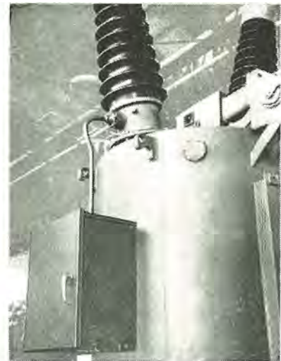
油入シャ断器に取付けた 154/\sqrt{3} kV 45 VA PBA-1 形 PD Type PBA-1 condenser bushing potential device mounted on breaker tank.
