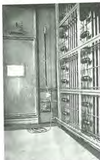
図 3.3 外被わく内面 (空気流入側) Fig. 3.3 Interior of cleanaire (air flowing inside).
