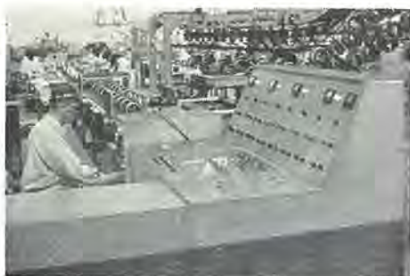
巻線試験装置 Coil testing device.
