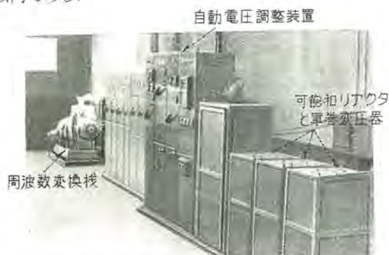
60 kVA 周波数変換機用静止型自動電圧調整器 Static automatic voltage regulator for frequency changer.
