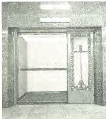
池袋三越納ギヤレスエレベータ乗場戸とカゴ室 Entrance doors and cab of D-C gearless elevators for Ikebukuro Mitsukoshi dept. store in Tokyo.
