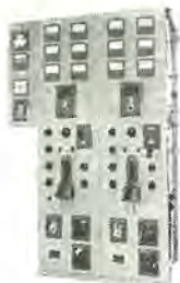
2×75 kVA 3,300 V 60 c/s 3φ 奄美大島納常用電源設備 用発電機盤 Generator panel for normal use power supply generator.
