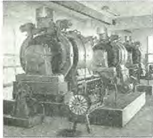
池袋三越納ギヤレスエレベータ巻上機 1,800 kg, 106 m/min D-C gearless traction machines 1,800 kg, 106 m/min for Ikebukuro Mitsukoshi dept. store in Tokyo.
