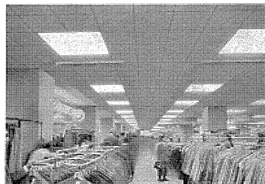
12 図 3～6 階売場埋込器具 Fig. 12. Flush mounted fixtures at 3rd～6th floor.
