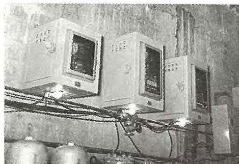
13 図 圧油槽油圧変換器、圧油槽油面変換器、水車流量変換器 Fig. 13. Converters for oil pressure, oil level of pressure tank, and water flow of turbine.
