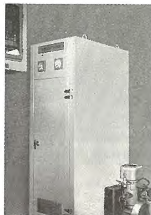
14 図 封水ポンプ制御盤 Fig. 14. Air compressor control cubicle for sealing water main inlet valve.
