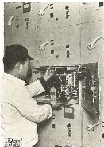
Fig. 6. Control center unit mounting.
