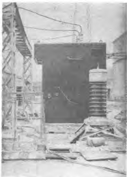
20-C-100 型空気遮断器内蔵屋外キュービクル View of 20 kV outdoor cubicle, Hirakata Substation, Kansai Electric Power Co., containing type 20-C-100 air blow circuit breaker.
