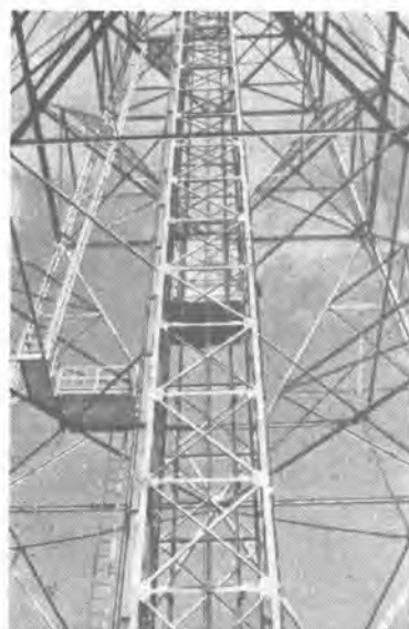
日本テレビ塔エレベータ Highest rise elevator at Metropolis (74m) for Nihon Television Broad Casting tower.
