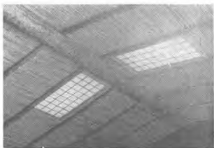
岩本楼の客室 Flush mounted fluorescent luminair at ceiling of Japanese style room.
