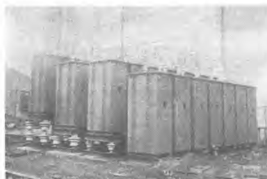
88 kV 10,000 kVA 60 \sim 蓄電器バンク Capacitor bank for charging current load.
