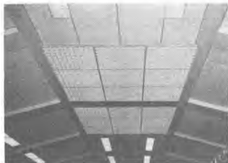
関西電力枚方変電所配電盤室照明 Fluorescent luminaires for control room.
