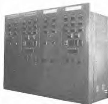
主配電盤計器面 Main switch board for synchronous condenser
